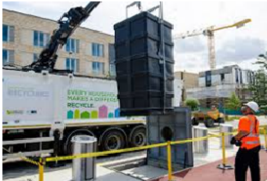
Top opening crane lift design at Eddington, Cambridge
