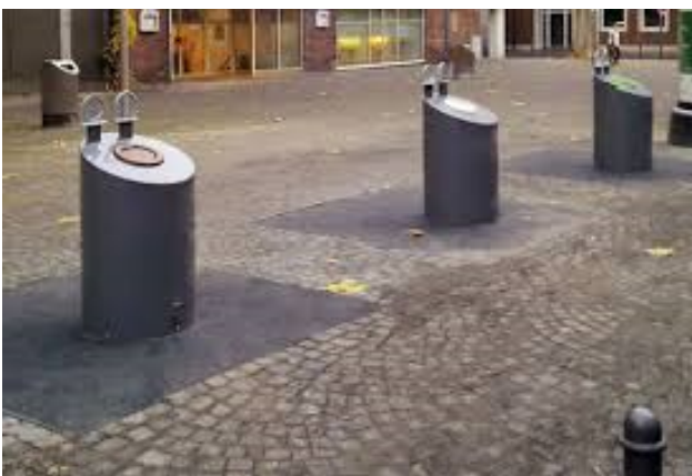
An example of underground waste storage
