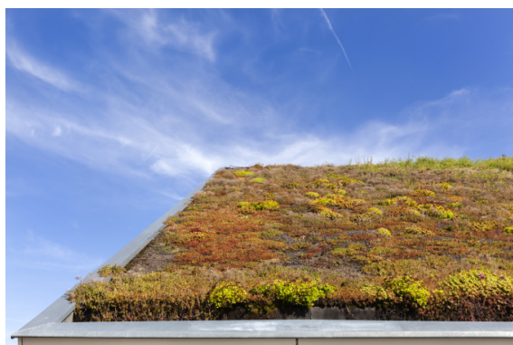
An example of an extensive green roof, which requires little management
